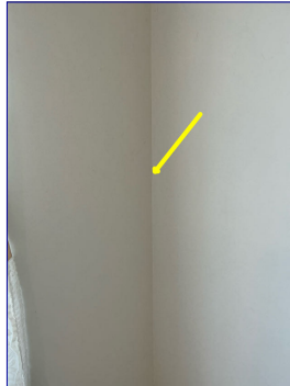
Small crack in the northeast corner wall of the family room area. Recommend monitoring and repairing as needed.
