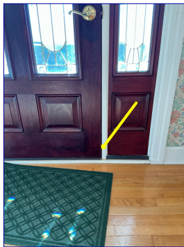
Area at bottom of front door where air is able to enter the home. Recommend contractor make necessary repairs.
