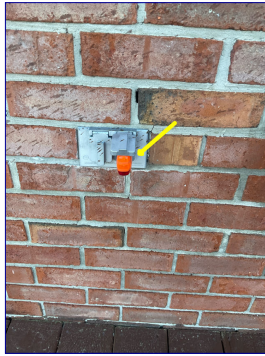
Exterior receptacle at deck area is not protected. Recommend electrician evaluate and make necessary repairs for GFI protection.
