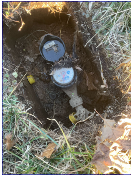
Main water shut off is at water meter located at Southeast corner of property.
