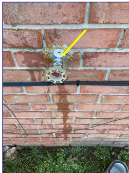
Frostproof hose bib at north side of house is leaking at the vacuum breaker. Recommend plumber repair leak and replace cap for vacuum breaker
