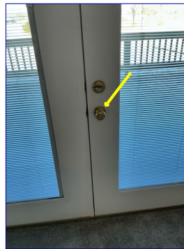
Unable to lock door handle of back door. Recommend contractor make necessary repairs.
