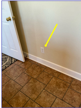
Loose receptacle in the kitchen area. Recommend electrician make necessary repairs.
