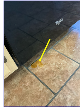
Leak at kitchen dishwasher door seal. Recommend plumber further evaluate and make necessary repairs.
