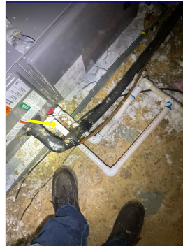
Recommend installing secondary drain safety switch for secondary drain port for HVAC unit in the attic. This will keep water from entering the draining pan if condensate trap for main drain becomes clogged. Recommend this be done at next HVAC service.
