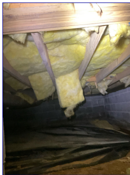
Insulation in the crawlspace is falling in some areas. Recommend having insulation placed back between floor joists.
